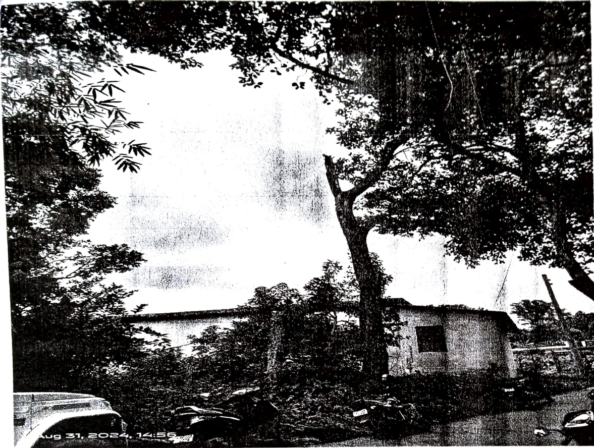
Picture 1: Fallen oie adjacent to road, parking area & green oie weakened by termites.
